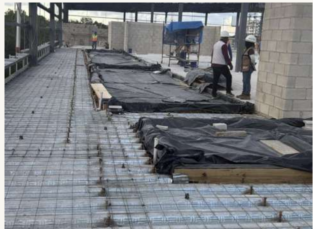
06 • Specialized formwork in cold storage areas
