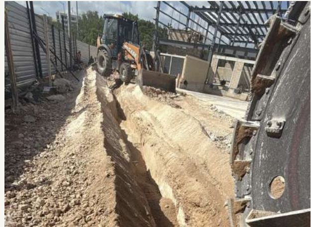
02 • Earthworks and high-capacity trenching
