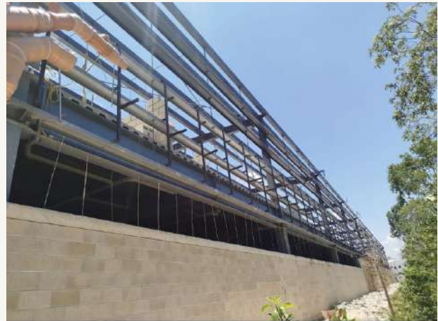
04 • Structural steel and roof erection
