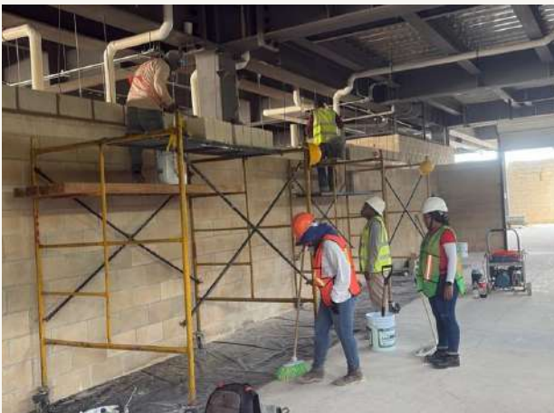
05 • Masonry and partitions
