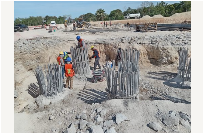
Works on deep foundation elements.
