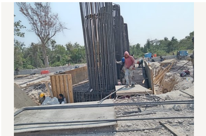
Formwork for foundation elements.
